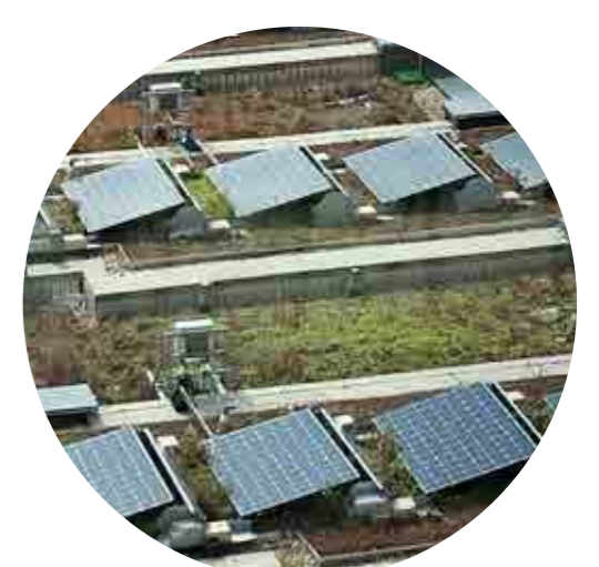
Solar Panels & brown roofs
