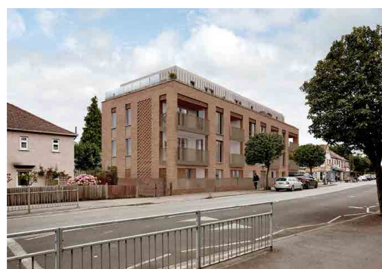
Mitcham, London Borough of Merton - Under construction. 14 apartments
