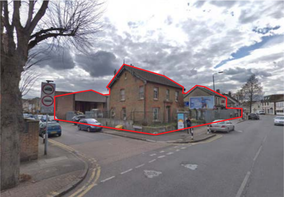
4 - View of the existing office units on site
