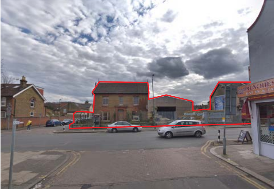
5 - View of the existing office units and merchant's warehouse on site
